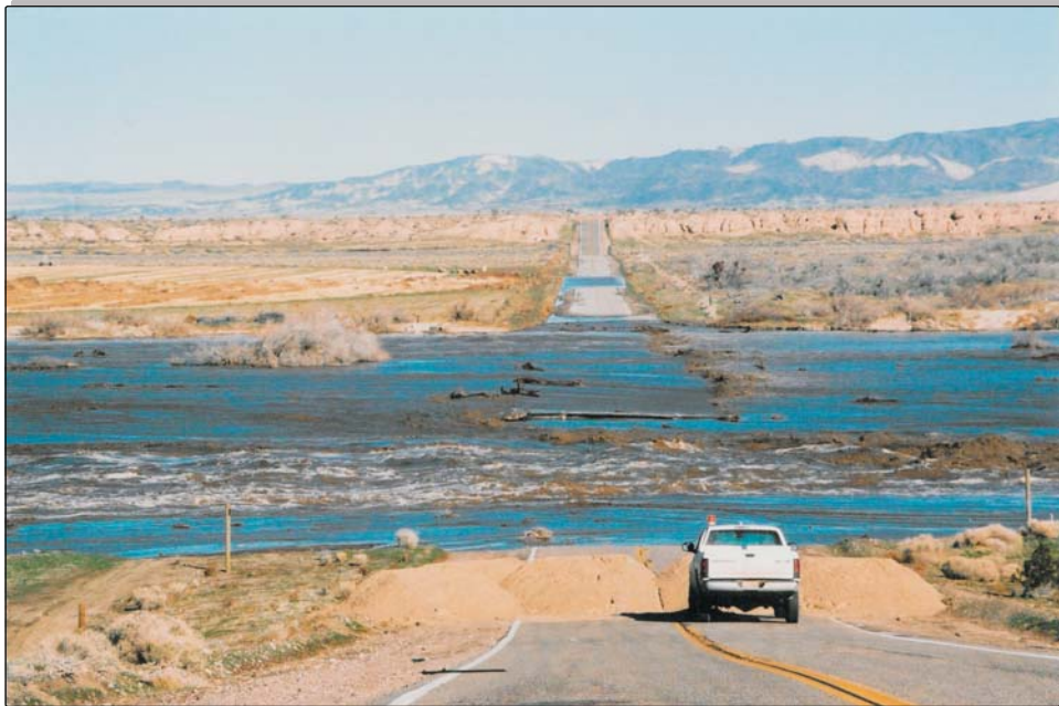
2005 Flood - Harvard Road crossing looking north
