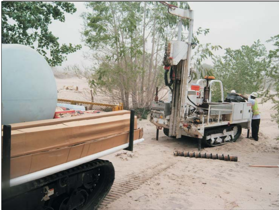
Hollow Stem Auger rig at Shallow Piezometer P6
