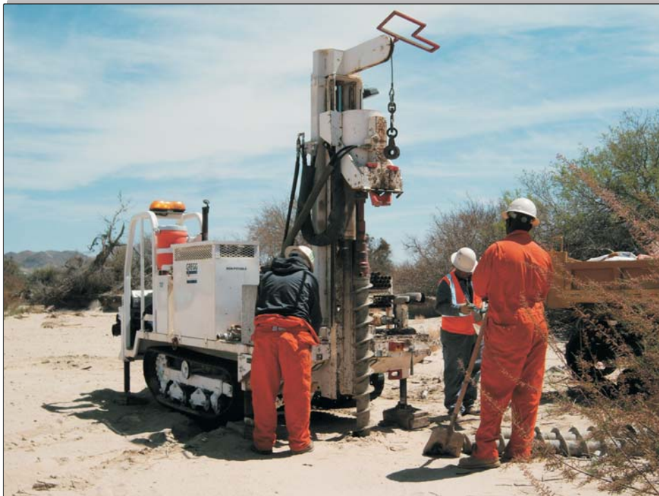
Hollow Stem Auger rig at Shallow Piezometer P4
