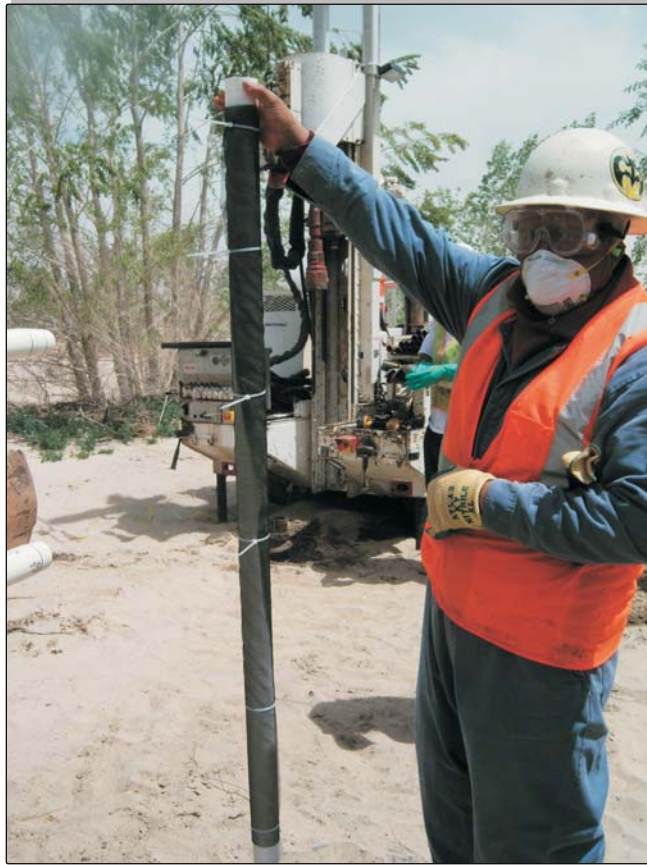
Well screen installation
